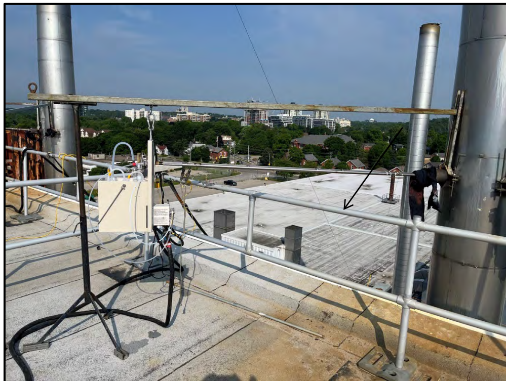
Figure B2: T105 East Furnace Stack (Typical of Both)
